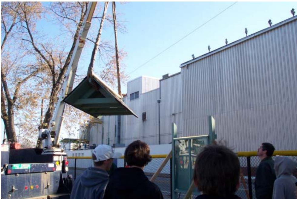
Figure 26 – Lowering roof onto kiosk via cherry picker
